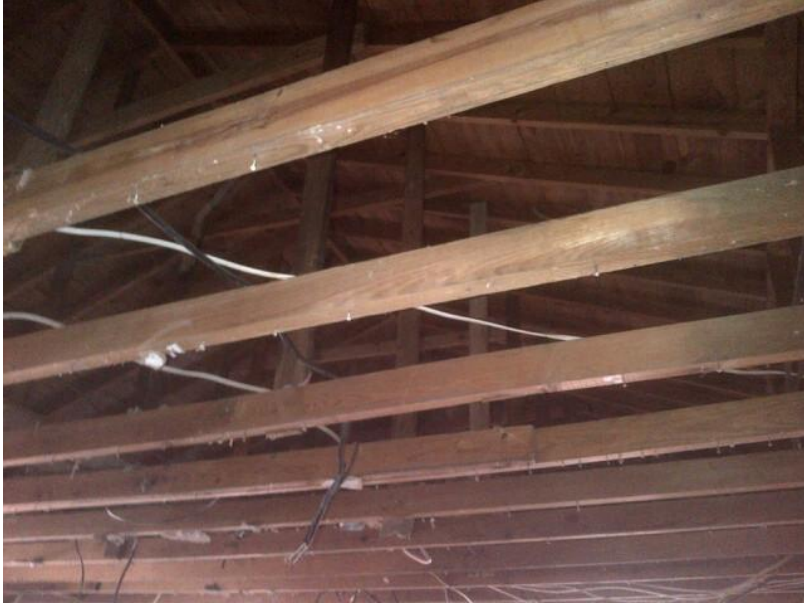
With the ceiling removed the attic and roof exposed
